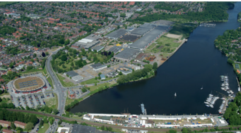
Headquarters of the ACO Group in Rendsburg/Büdelndorf, Germany
