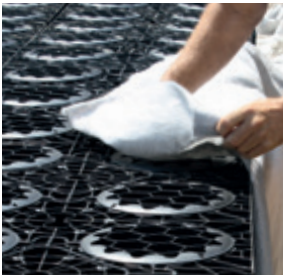
The protective geotextile is then laid around the infiltration system so that it is completely covered
