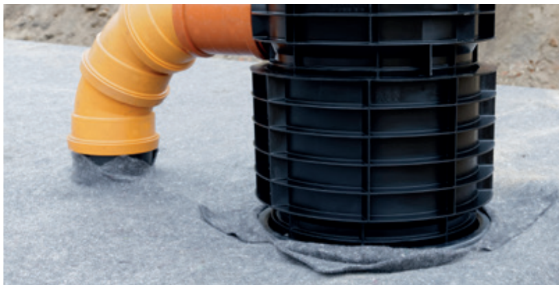
The geotextile is cut in and is pushed over the pipe adapter
