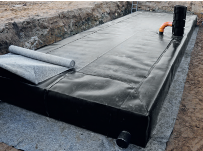
The outer protective fleece is applied once the sealing membrane is complete
