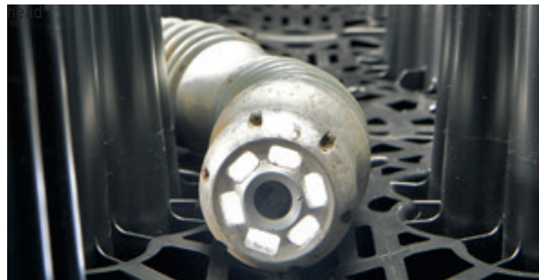
Push camera, cleaning equipment with a rinsing
