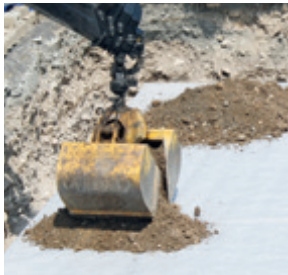
Filling the infiltration system
