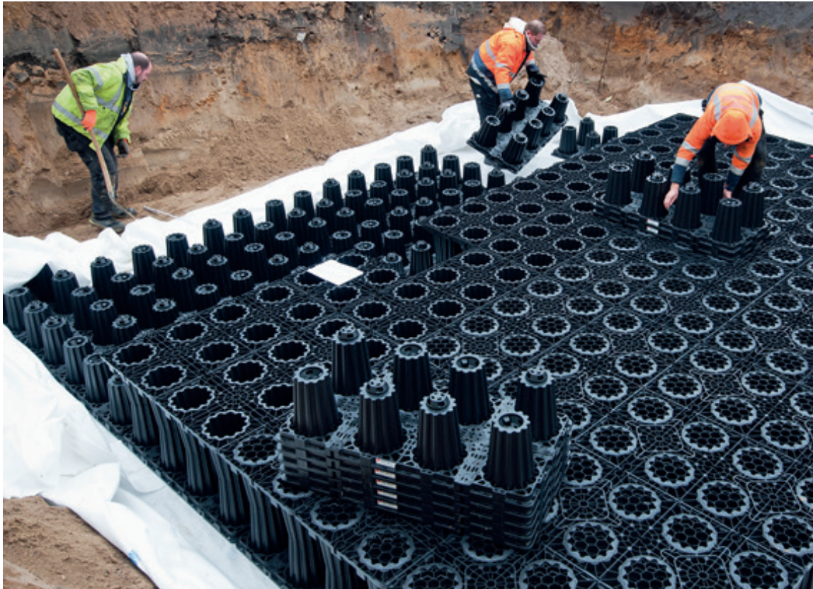
ACO Application Technology creates a corresponding installation plan for every building project. Reference project: Heider Marktpassage, Heide: ACO Stormbrixx HD as an infiltration system underneath car parking areas.
