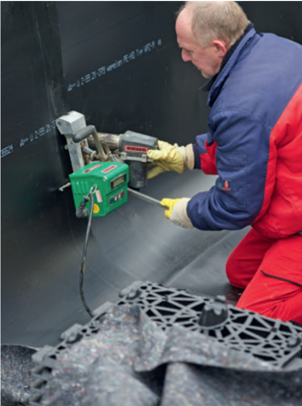
The sealing membrane is then welded
