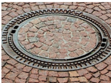
Shaft cover in the block paving surface
