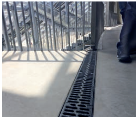
ACO DRAIN® Multiline Seal in for all-round use in the stadium
